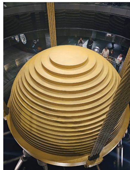
The stabilizing ball in the Taipei 101. It helps to hold the building steady in an earthquake.
